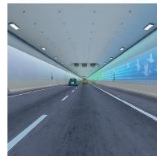
Fehmarnbelt Fixed Link Tunnel, Denmark - Germany
