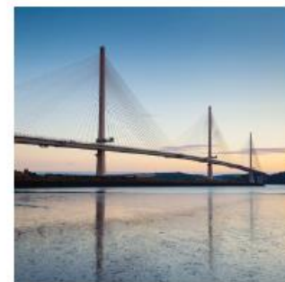
Queensferry Crossing, Edinburgh, UK
